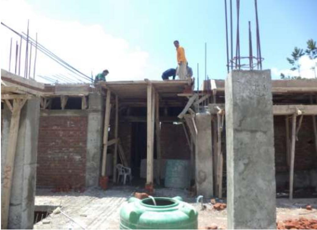
(Right Wing) - Scaffolding work for laying of slab of first floor underway
