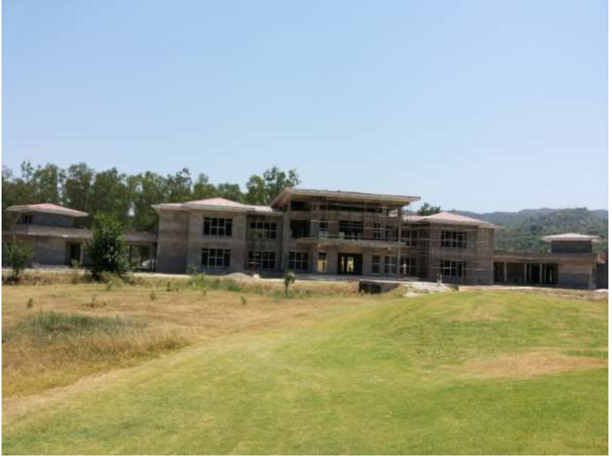
View of Club Building from Golf Course
